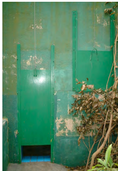
Sliding door design controlled outside the cage
