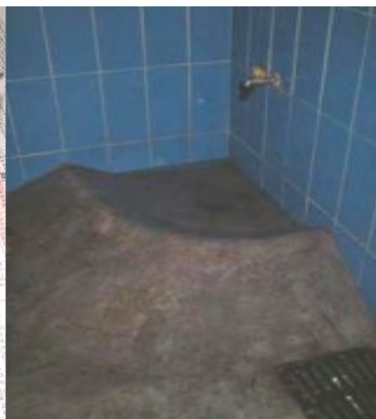
A built in smooth concrete drinking trough with low gradient textured sides to allow easy access to the water source.
