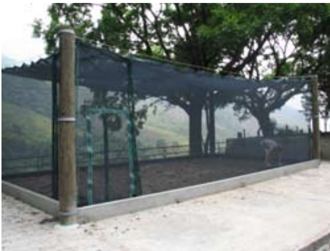
Newly completed WARC Flight Test Enclosure.
