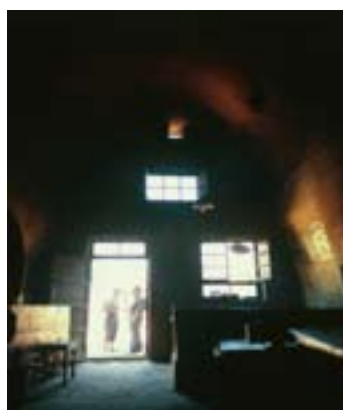
Poor ventilation, limited space and insufficient lighting are common problems of traditional earth-built housing at Gansu.
