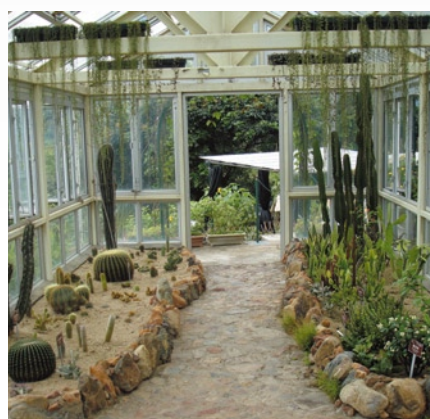
Outlook of the Cactus Greenhouse after renovation.
