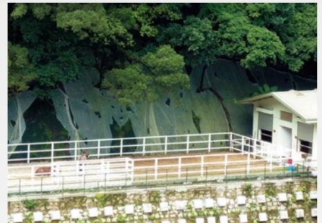
Stabilization of slope behind Mule Stables.
