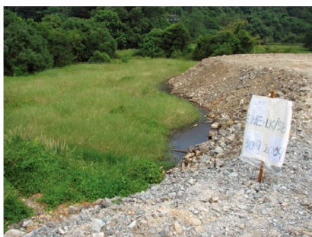
Illegal filling of ponds with construction and demolition wastes at Luk Keng, North East New Territories.
