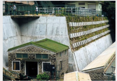
Stabilization of slope behind the Chicken Houses.
