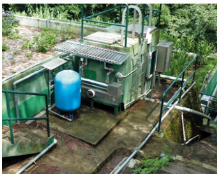
Sterilization system for re-circulation of treated waste water.
