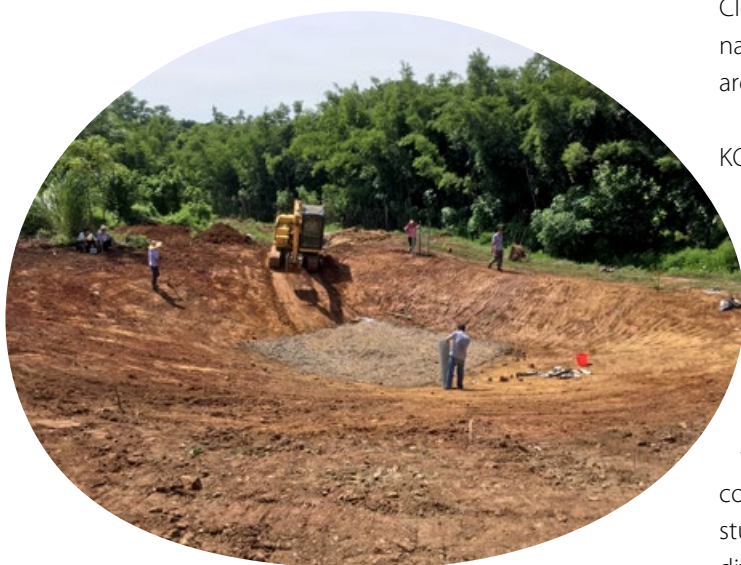
A waterhole with waterproof lining, designed by KCC, in Bangxi Nature Reserve, Hainan being constructed to provide freshwater for the Eld's Deer during the dry season.
