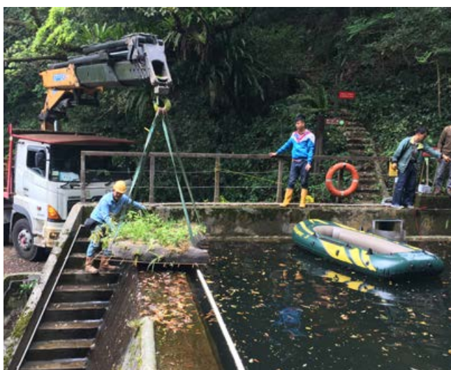
● Installation of one of the two floating islands at Magnolia Reservoir.
