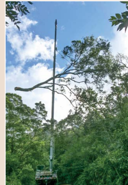
Removal of two very large Acacia confusa trees by crane
