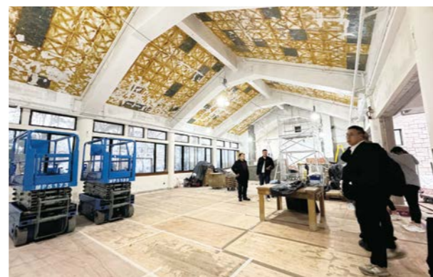
Renovation work at the Food Hub
