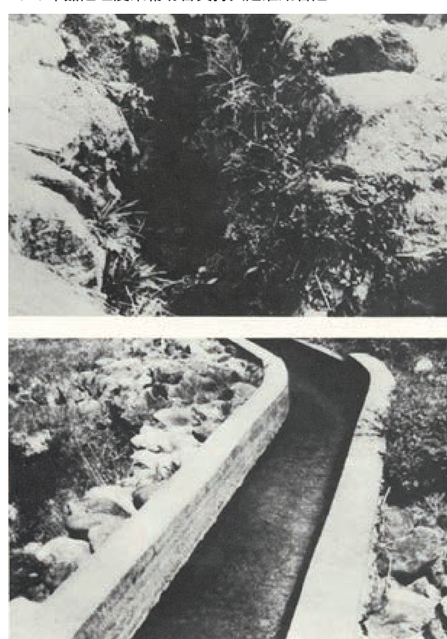
Improved irrigation channel 改良後之灌溉管道
